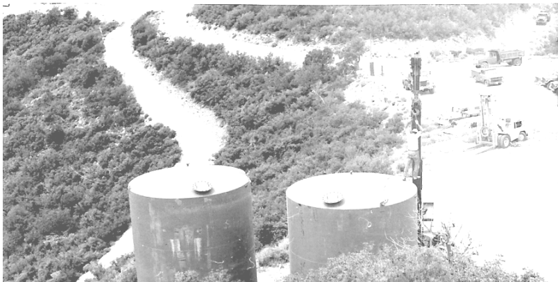
RIDGE WATER TANKS INSTALLATION BY SUPPORT GROUP October 10, 1976
