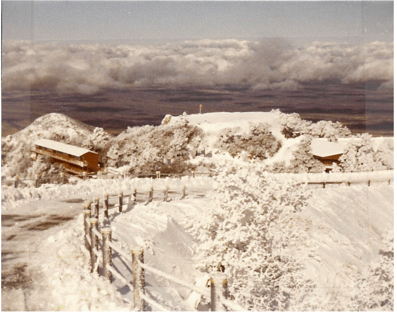
BOWL DOMITORY LOOKING DOWN FROM THE HEATED CONCRETE ROAD
